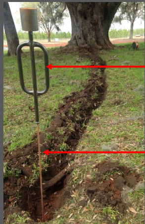
Ground Rod Installation
