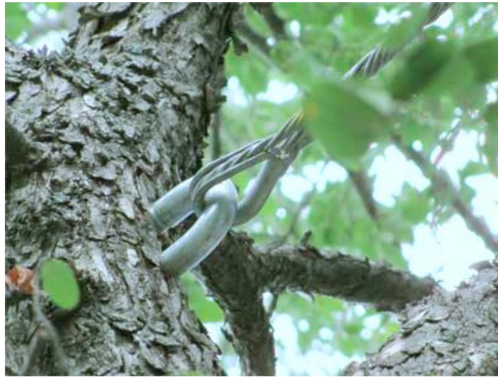
A cable and lag hook installed
