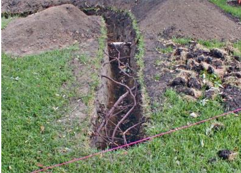
Using compressed air as a “shovel” preserves lateral roots and allows for irrigation lines and other utilities to be installed under spreading root systems. Photo by Bill Seaman
